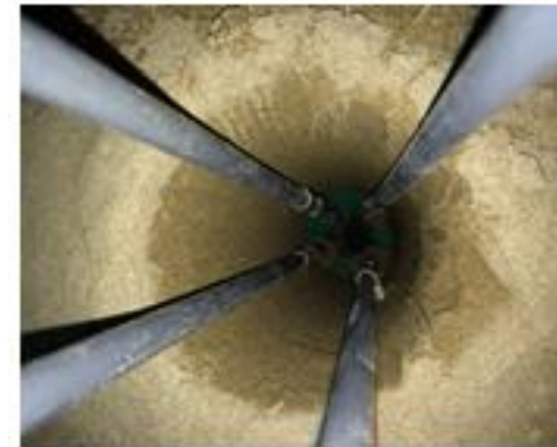
Shaft post-grouted precast-in-place pile
